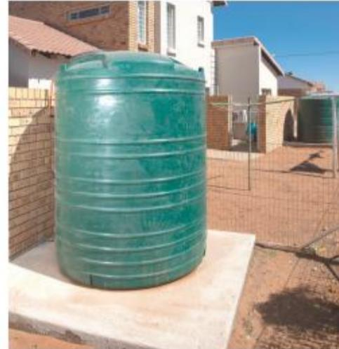
The water tanks have a capacity of 2,500 litres each, with an accompanying pressure pump on a newly casted concrete base.
