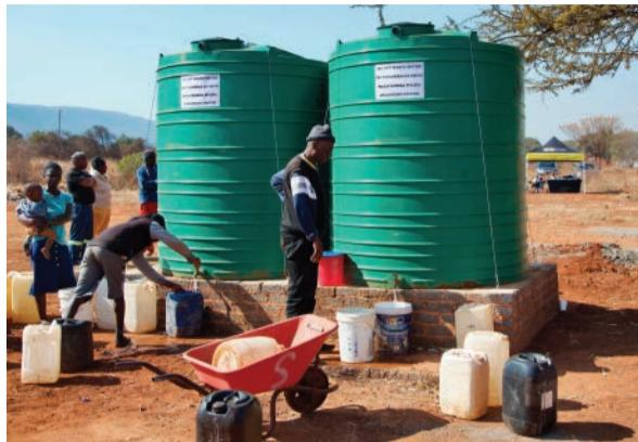
This system pumps 1 600 litres of water per hour to the storage tanks to supply water to 3 000 African households.
