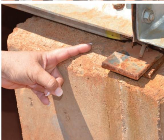
A finger pointing out the correct position of where the reservoir's joints should have rested.
