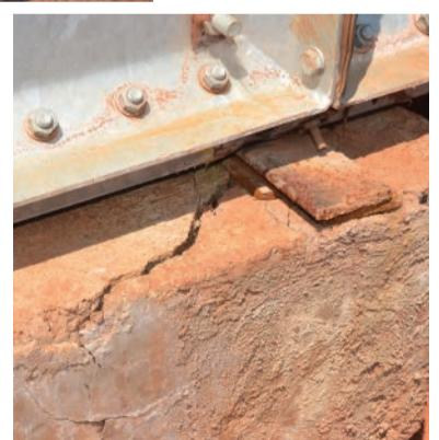
The result of incorrect positioning of the Tierkloof reservoir's panel joints. This could eventually see the reservoir collapsing and flooding large areas of Schoongesicht.
